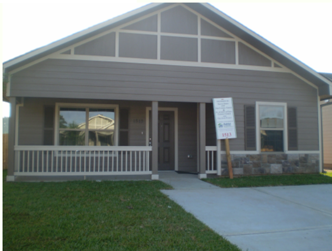
Front of the Completed 3-Bedroom Home
